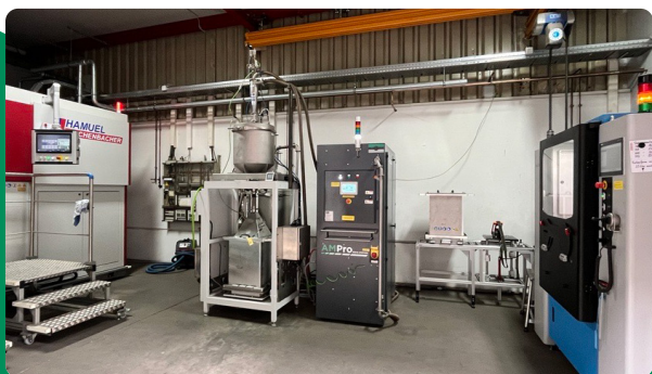
The Russell AMPro® Sieve Station installation
