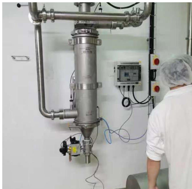
图2：Self-Cleaning Russell Eco Filter®自清洁式过滤器的安装
